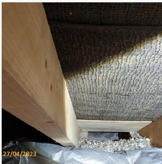
Vermiculite insulation to the centre beam
