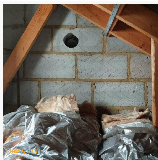
Ventilation required in the roof void
